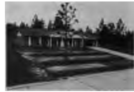
Figure 6 An example of bench leveling to prevent erosion in an urban area.
